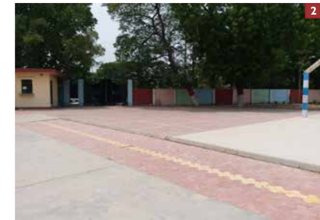
Space for staff car park within the school premises
