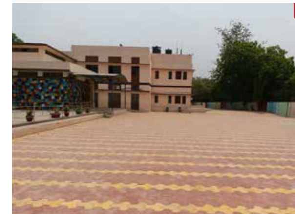
Space for staff car park within the school premises
